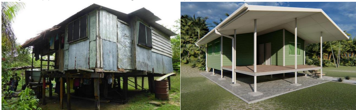
Figure 9: (A) House in Woodlark mining lease area and (B) new house design for those moved under the RAP
